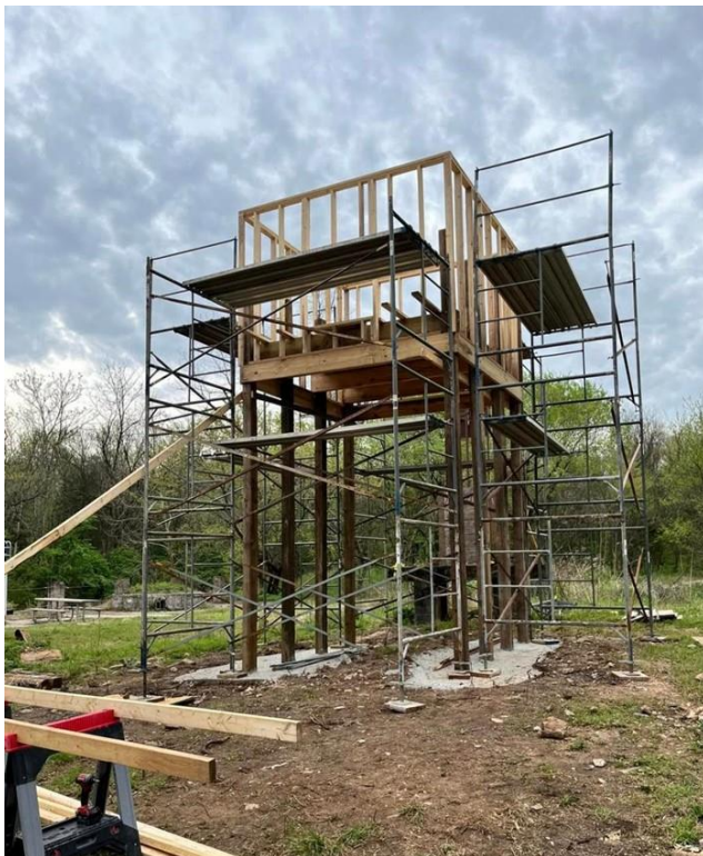
The Ijams bat house during the early phase of construction in spring 2025.
